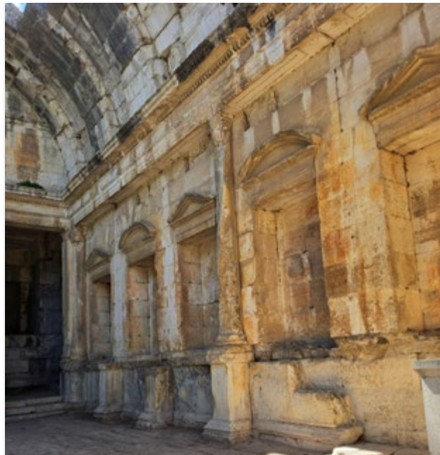
©Photos : Pwatrik Koune
